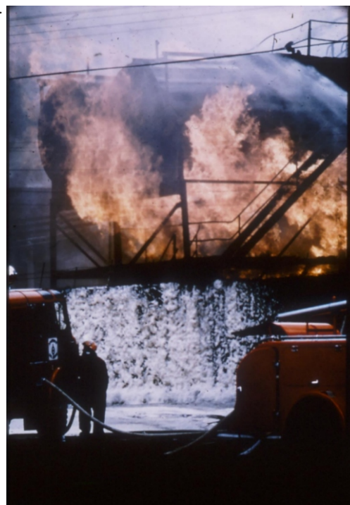
Below: The foam that proved to be useless runs down the front of the retaining wall surrounding the terminal. Note the firemen still on the top of the large tanks.
