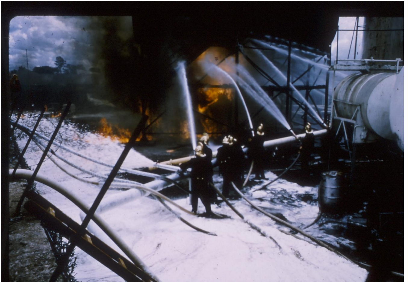
Below: A wonderful photo showing five lines of canvas trying to extinguish the flames up high, plus a foam cannon being used to try and douse the flames on the ground caused by the fuel run off.
